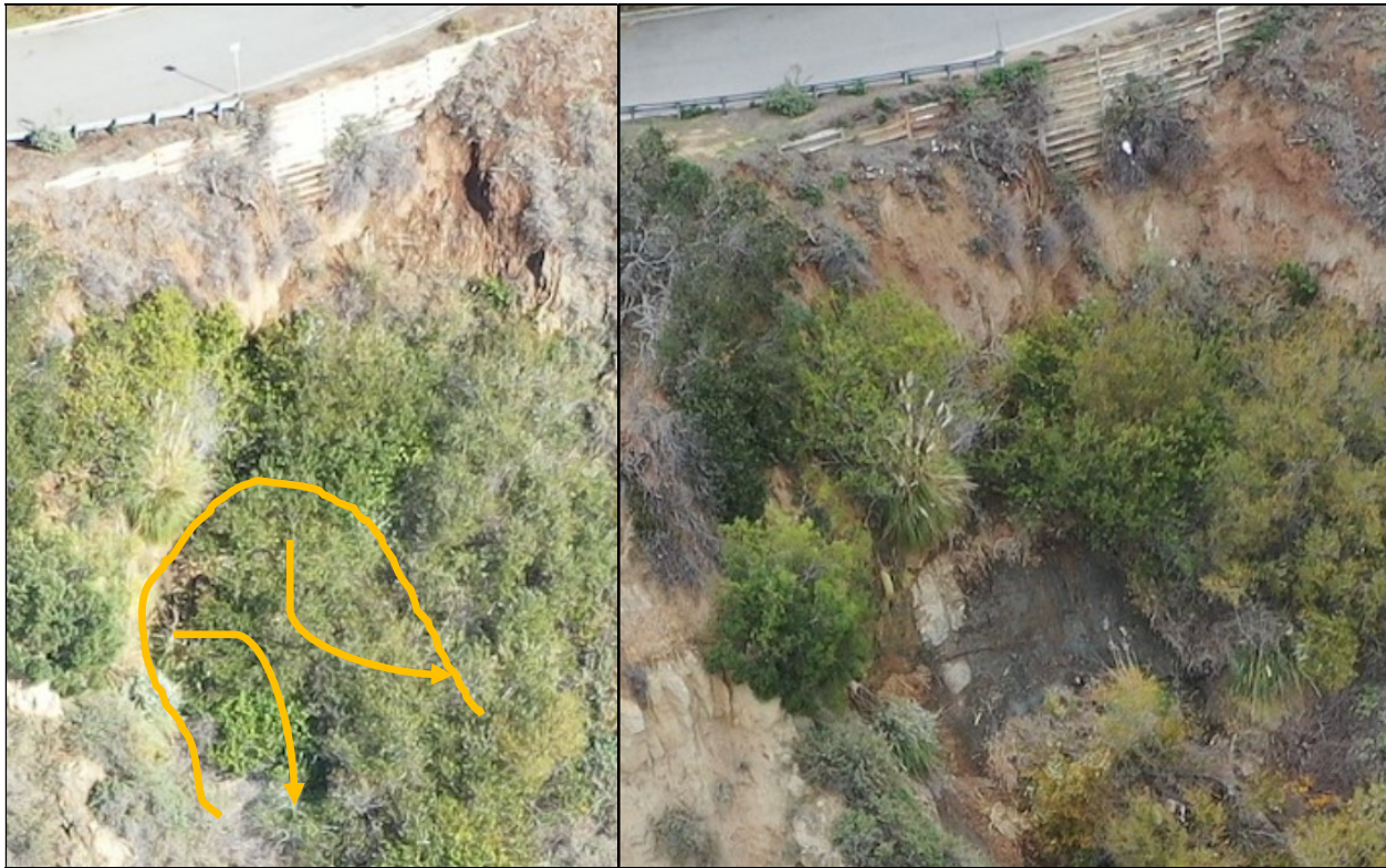
Photo 1: Photo on the left is of December 2021 before the slide occurred, and photo on the right is from January 2022 following the slide. The yellow outline illustrates the approximate limits of the slide on the before picture.
