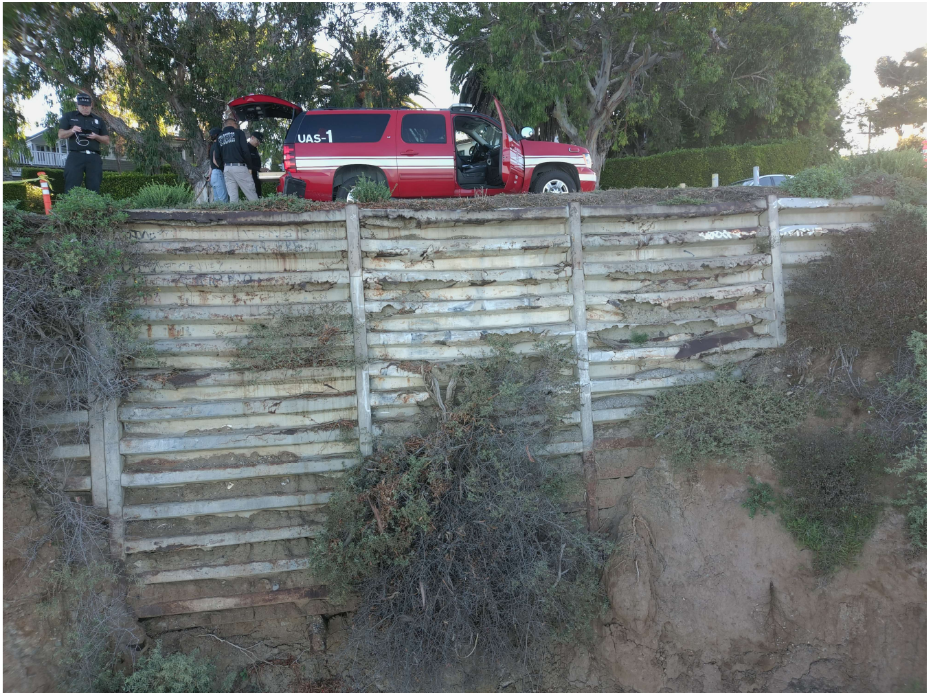
Photo 3: The deteriorated state of the ribbed-metal bulkhead. The soil in front of the bulkhead looks to have sloughed off, the date of which it occurred is unknown, and the base of the bulkhead looks to be slightly undermined. The bulkhead also has roots that have broken through the corroded face of the bulkhead.
