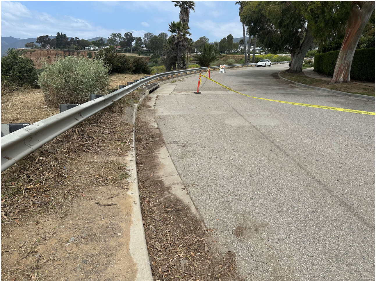
Photo 4: No tension cracks are observed to be affecting on the street, and the storm drain system and the northern end of the in-place bulkhead does not show any signs of damage or water buildup. As the drain appears dry, it does not appear likely that the water emanating on the slope is a result of a leaking storm drainpipe.
