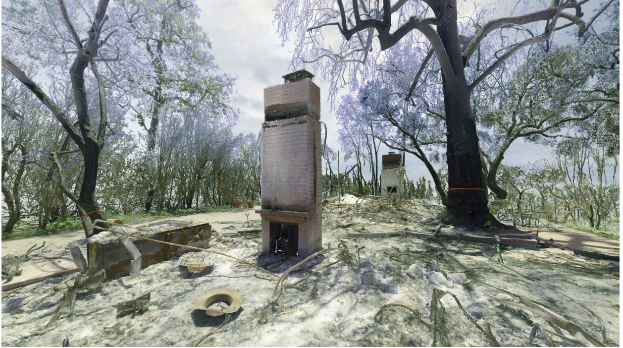
3D Point Cloud of an Eric Lloyd Wright chimney. Captured by AQYER, LLC.
